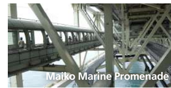
Akashi Kaikyo Bridge
